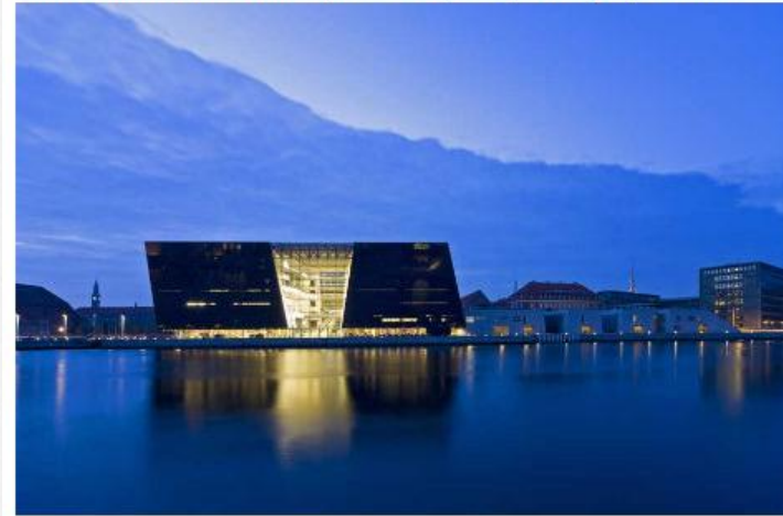
Black Diamond at the Royal Library Copenhagen, Denmark
